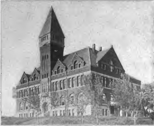
MAIN BUILDING, FAIRMOUNT COLLEGE.
